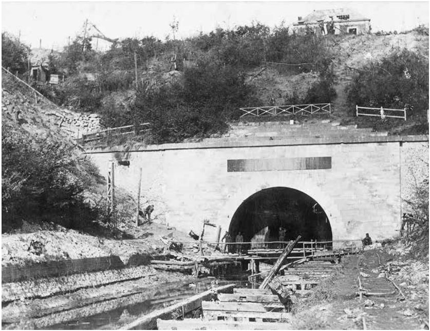
Entrance to St. Quentin Canal tunnel near Bellicourt, France (National Archives)
