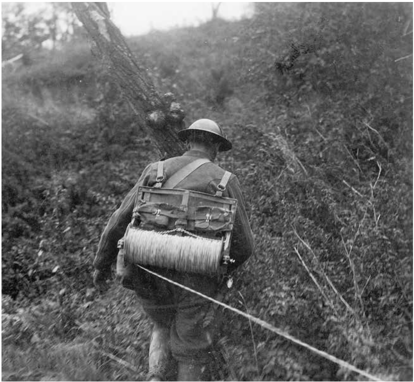
Member of the 101st Field Signal Battalion stringing telegraph wire in captured German position (National Archives)
