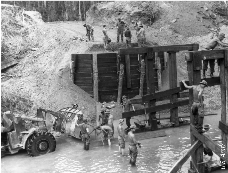
Bridge under construction along Route 547
