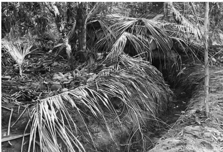
Coconut log bunker with fire trench entrance in the Buna Village area. (DA photograph)
