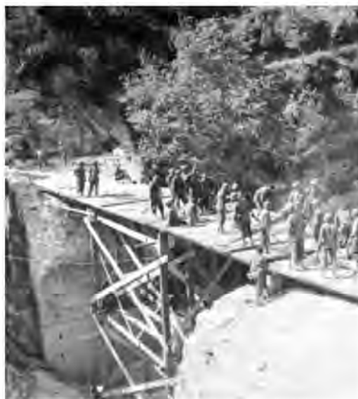
ENGINEERS REPAIRING A BRIDGE NEAR ACERNO
