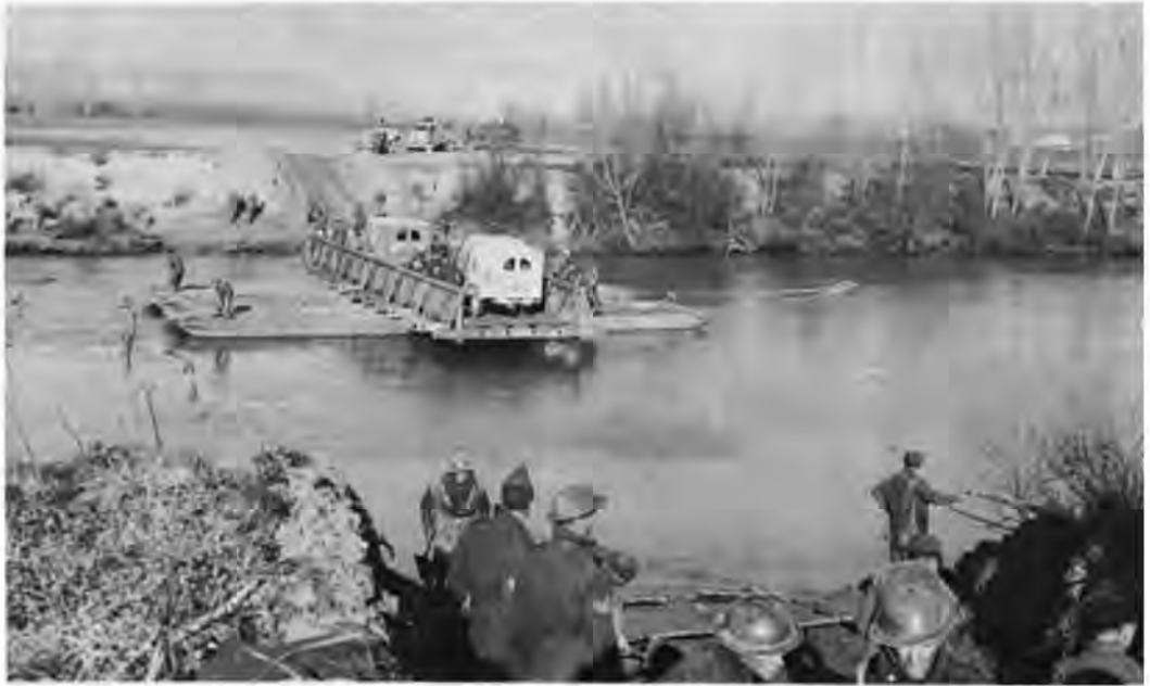
BRITISH 10 CORPS TROOPS SHUTTLING AMBULANCES ACROSS THE GARIGLIANO on a Bailey ponton raft.
