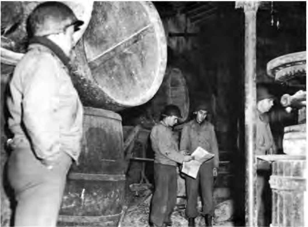
WINE CELLAR THAT SERVED AS VI CORPS HEADQUARTERS
