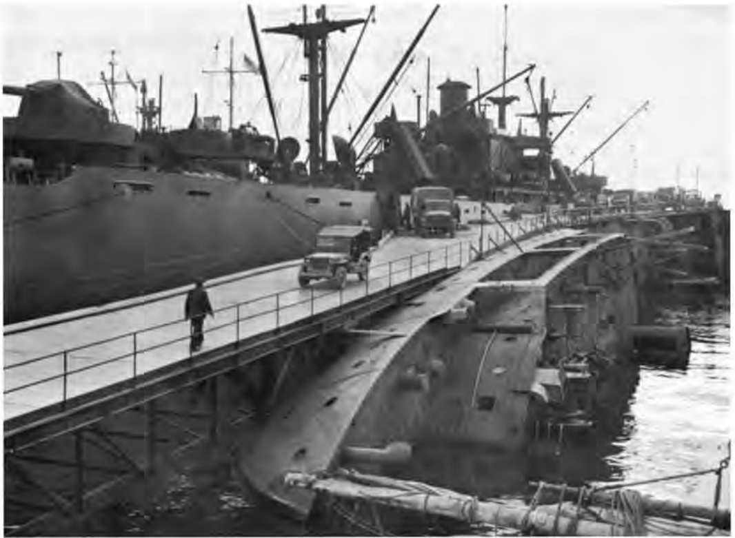
PIER BUILT ACROSS THE HULL OF A SUNKEN SHIP, NAPLES
