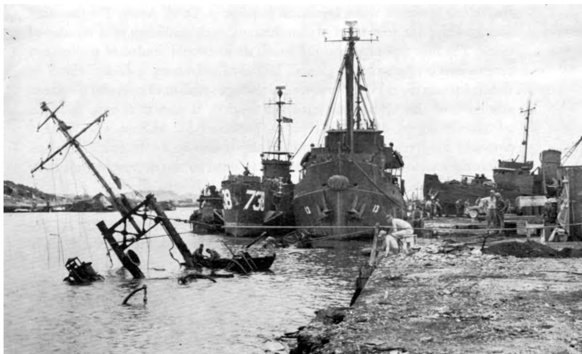
REHABILITATION OF PORT at Naha was in progress when this picture was taken, 19 June 1945.
