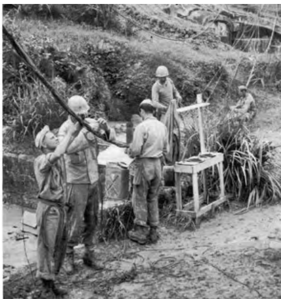
Main west-coast telephone cable
