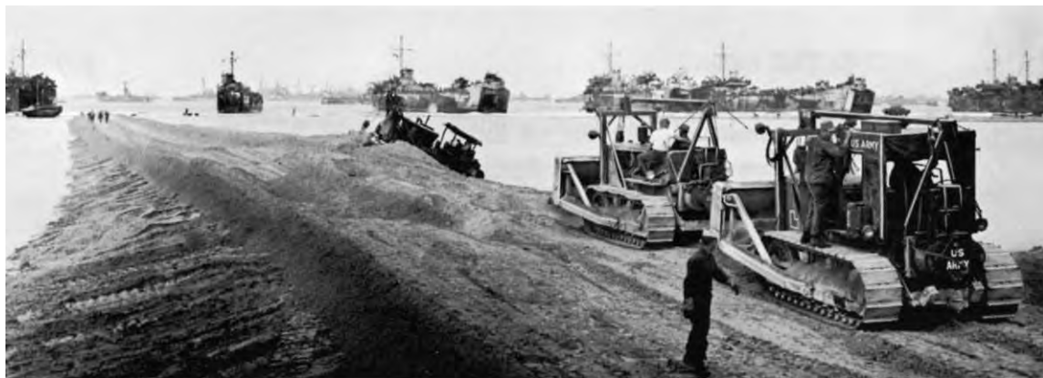
Ship-to-shore supply causeway at Hagushi beaches
