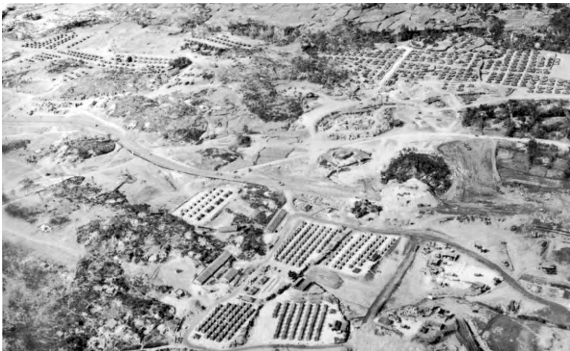
Large supply installation in Kakazu area
