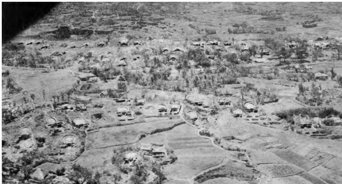
OKINAWAN CUSTOMS include the burial tomb and the veneration of ancestors. The burial tombs characteristic of the Okinawan landscape stand out clearly in this aerial view (above) just north of Shuri.
