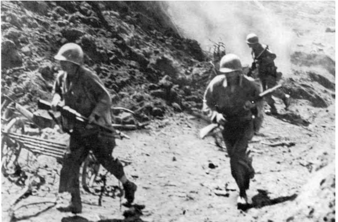
CORKSCREW— demolition team runs from cave blast.
