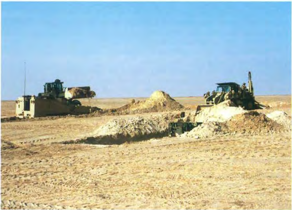
Small Emplacement Excavator; below, Small Emplacement Excavator and Armored Combat Earthmover (Left) Used To Dig Protective Positions for Vehicles and Equipment
