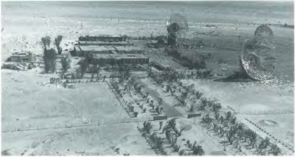
Damaged Iraqi Radar Facility
