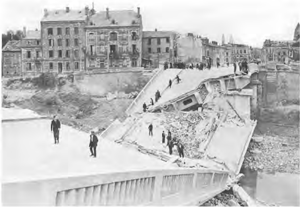
DEMOLISHED BRIDGE AT CHÂLONS-SUR-MARNE
