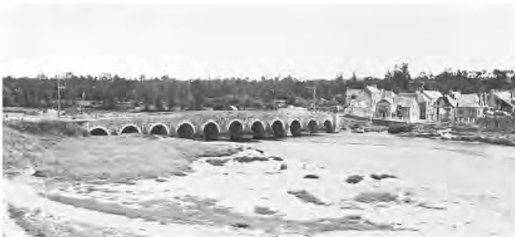
PONTAUBAULT BRIDGE over the Selune River, one of the few bridges left intact by retreating Germans.
