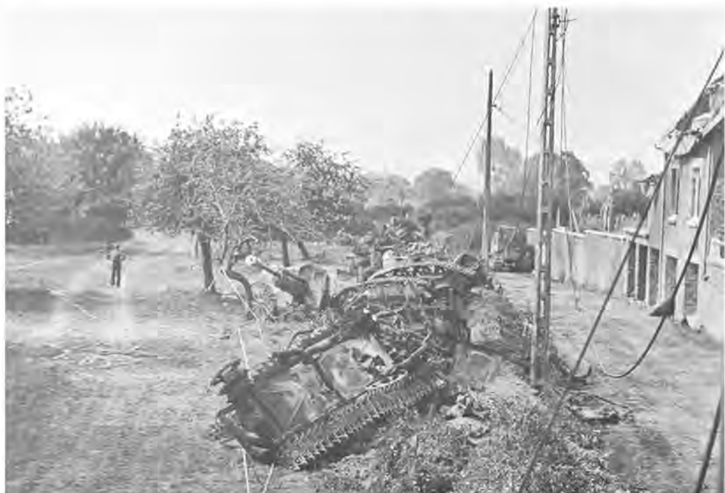
WRECKED GERMAN ARMOR BULLDOZED OFF A ROAD NEAR RONCEY
